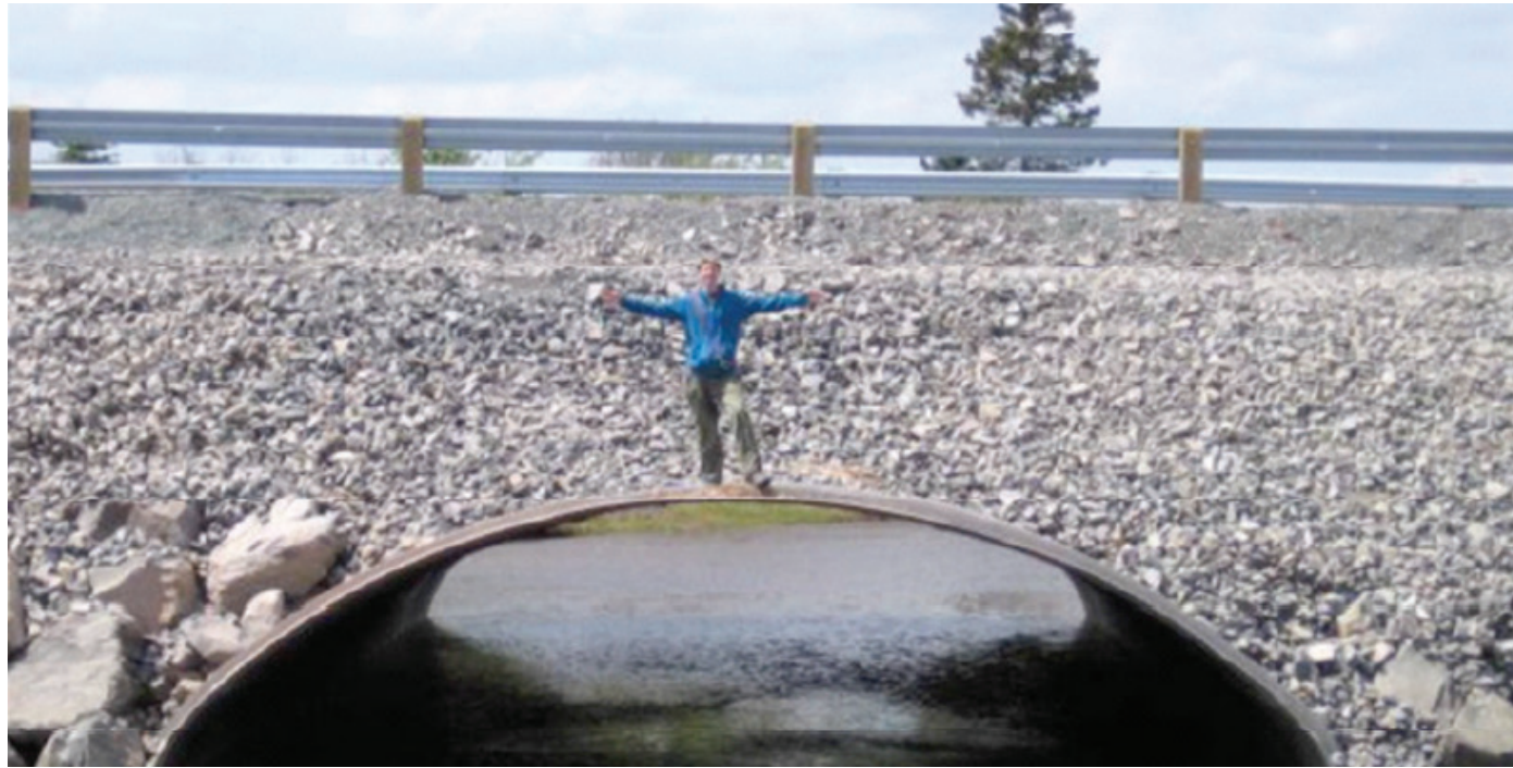
Figure 9. The culvert installed in December 2005 for the restoration of the Cheverie Creek salt marsh. Photo credit: Nancy Neat 2006
