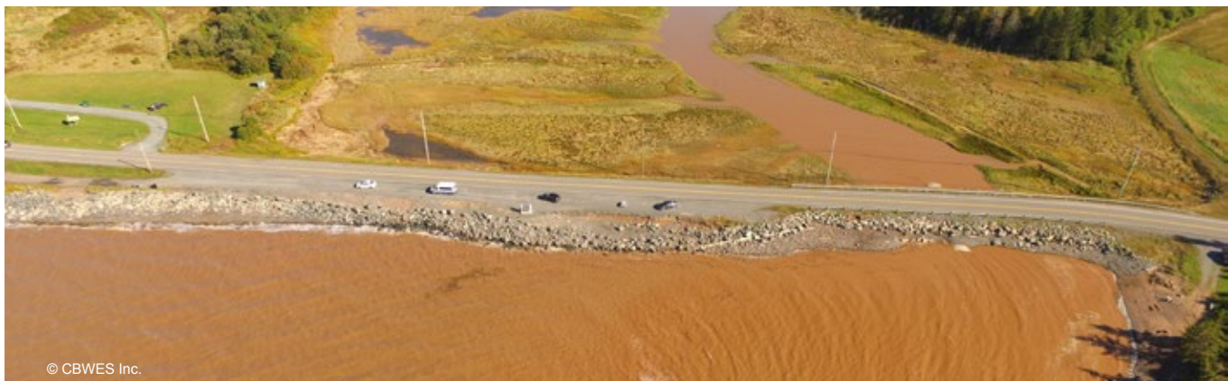
Photo: The Cheverie Creek, Nova Scotia, tidal river and salt marsh restoration project replaced an old wooden culvert in 2005, restoring tidal flow and fish passage to 43 hectares of tidal wetland habitat. The project included 7 years of post-restoration monitoring. Project partners include Nova Scotia Department of Transportation and Infrastructure Renewal, CBWES Inc., Saint Mary's University, DFO Small Craft Harbours, and the local community.
